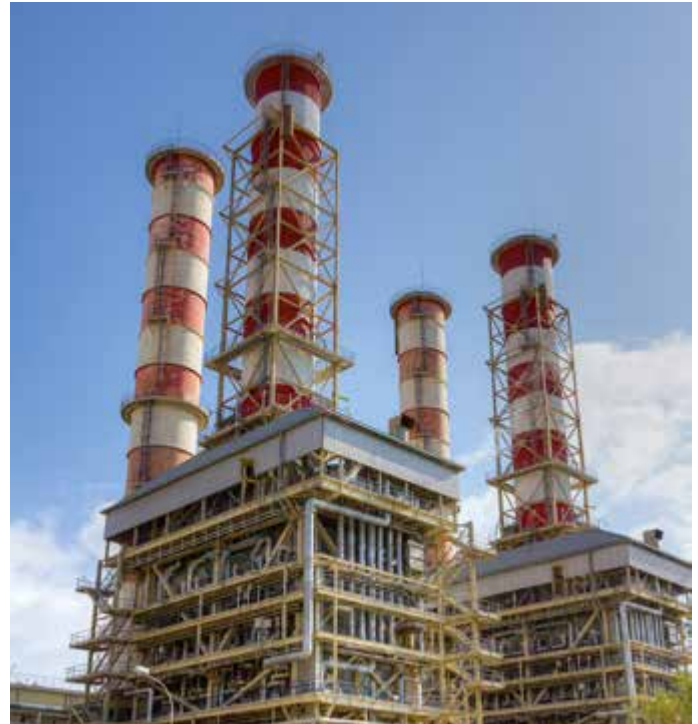
Sulzer was contacted to repair a 45 MW generator in a gas fired power station.
