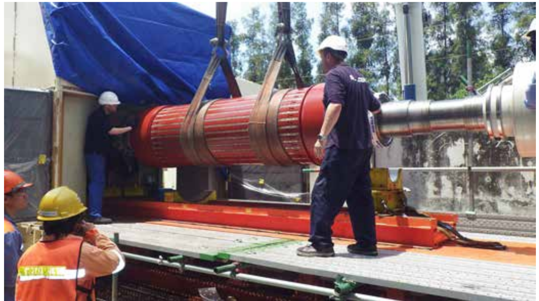
Sulzer used a 220-tonne mobile crane to lift the 12-tonne rotor.
