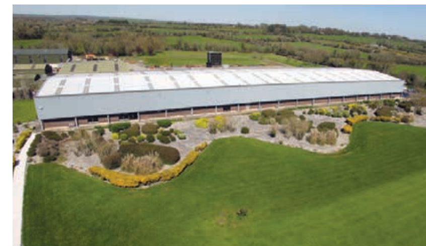
Aerial view of the premises.
