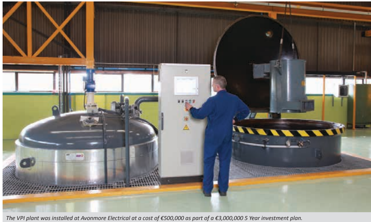
The VPI plant was installed at Avonmore Electrical at a cost of €500,000 as part of a €3,000,000 5 Year investment plan.
