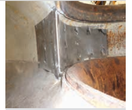
Volute Leading Edge Refurbishment.
