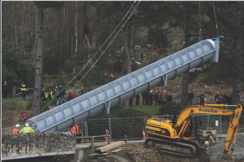
The new Archimedes screw being installed at Cragside in Northumberland
