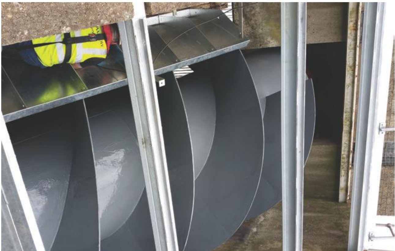
Installed Screw with New Channels and Deflectors
