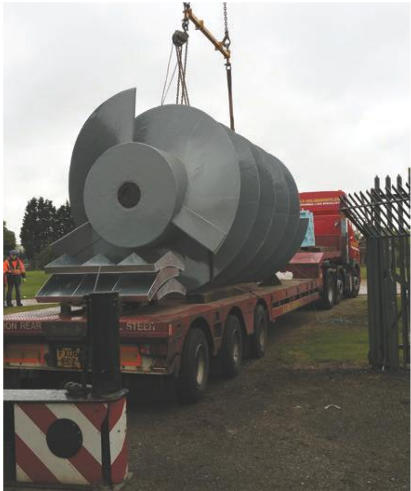
Ready to Lift On Site
