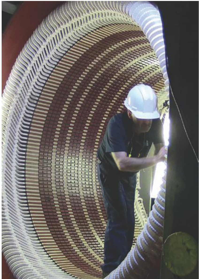
Houghton International coils in a power station diesel generator rewind, Central America
