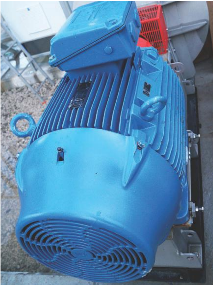
The centrifugal fans employ 175kW WEG W22 Premium Efficiency IP55 IE3 3~ electric motors. They are foot mounted to a skid and connected using a torque limiting anti-vibration coupling to the fan drive shaft.
