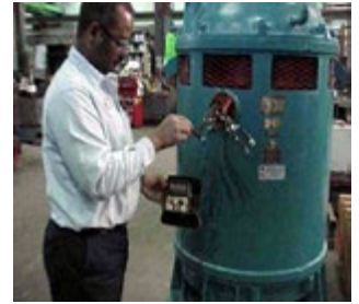
Figure 4. Use of a digital megohmmeter to check winding insulation resistance.
