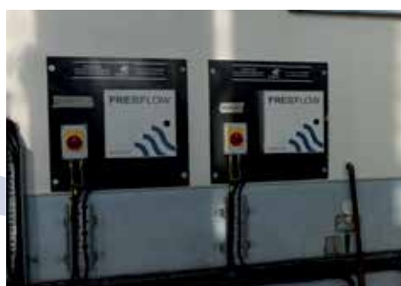
Figure 4 FREEFLOW Data Acquisition Unit (26 installed)
