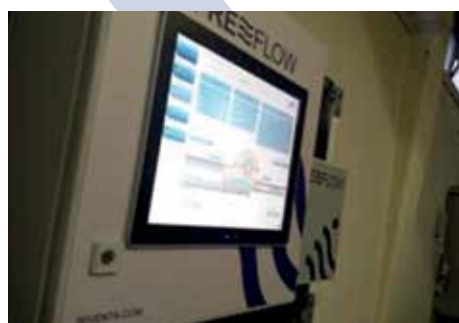
Figure 3 Human Machine Interface (HMI) (5 installed)
