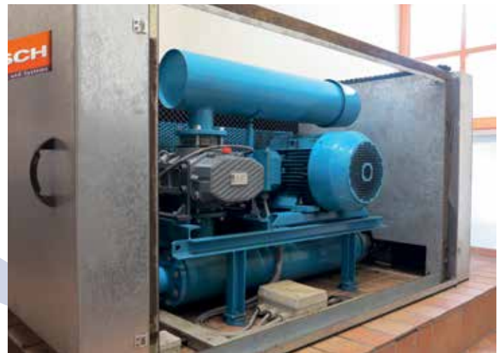
One of the two Busch Tyr blowers used for air injection into the aeration tanks
