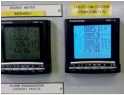
Figure 6 Electrical power metering (26 installed)
