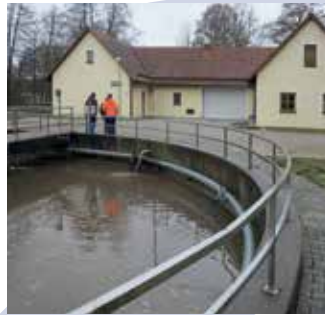
Sewage treatment plant operated by the Schlammersdorf-Vorbach waste water treatment authority
