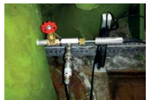
Figure 5 Hydraulic efficiency pressure and temperature transducers (104 installed)
