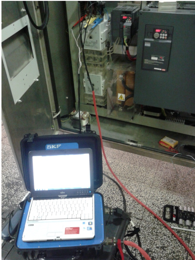
415v Inverter Driven
