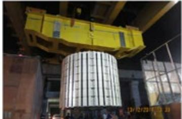
Installation of Rotor Rim Assembly of 333 MW Hydro Generator
