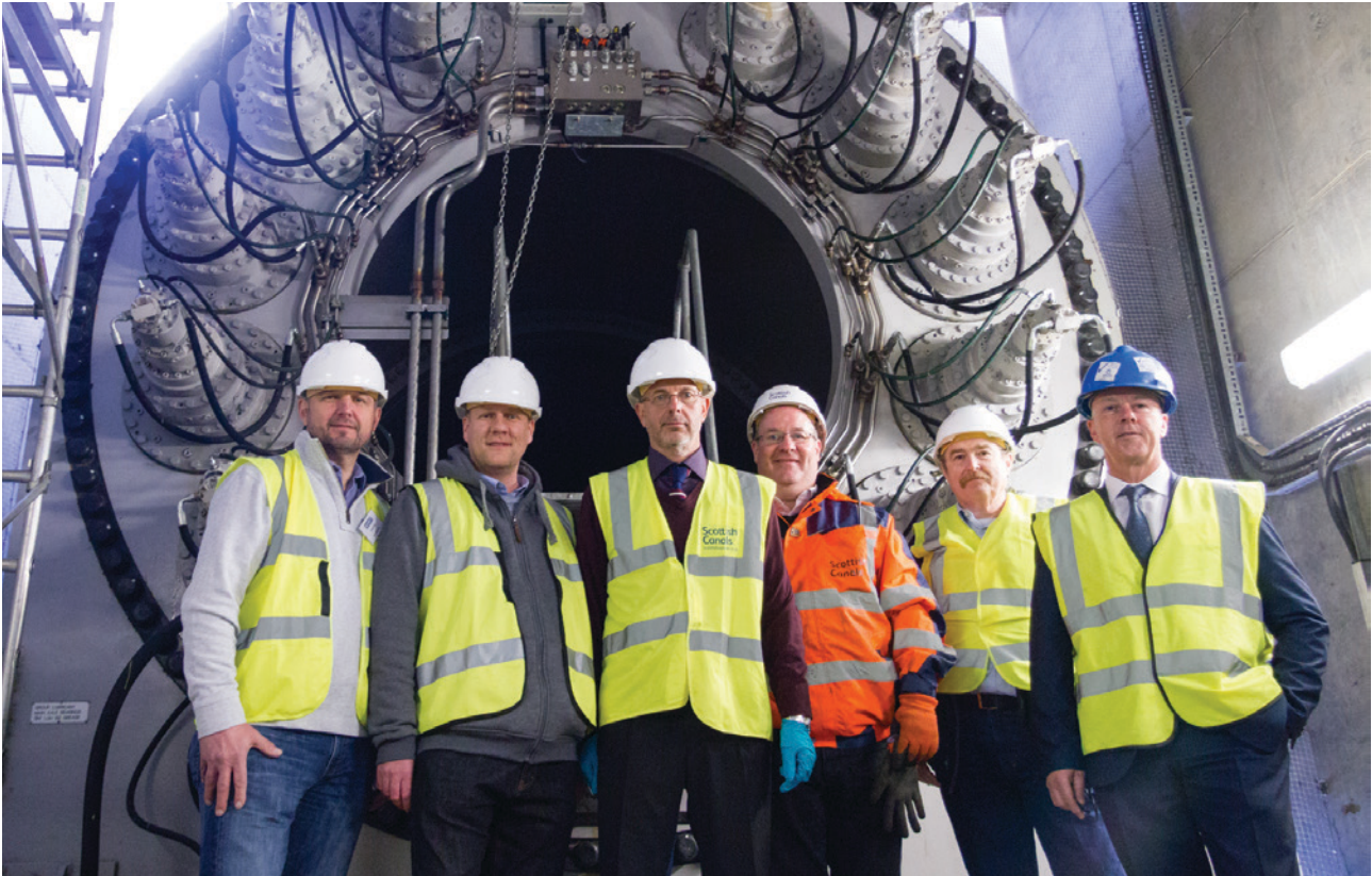
AEMT members were able to gain an exclusive audience with the Principal M&E Engineer for the Falkirk wheel then taken on a tour of the wheel's engine and maintenance rooms.
