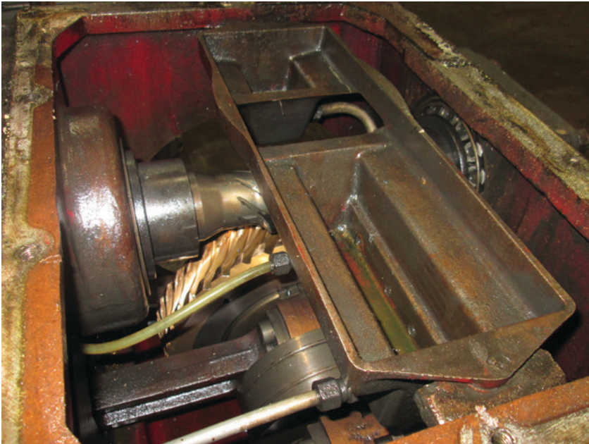
Fig 2. The pump internals were badly worn.
